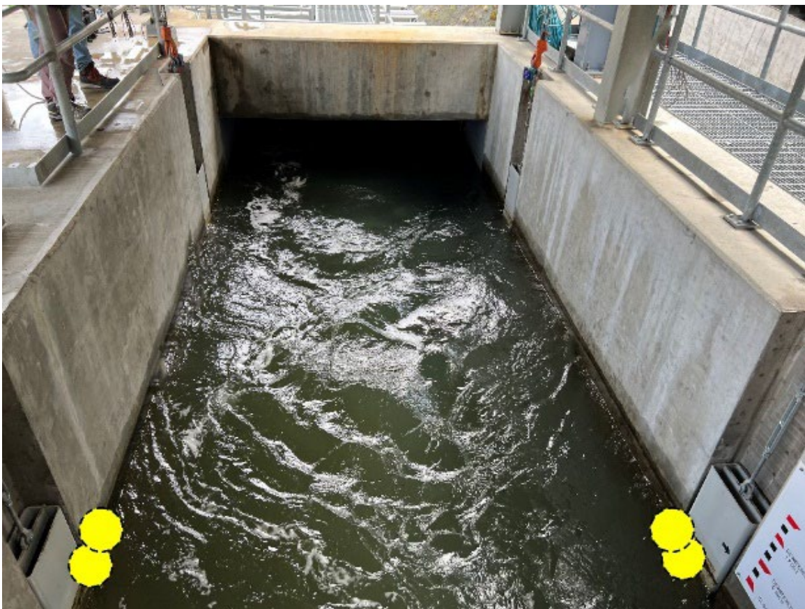
Figure 2. Location of the hydrophones at the downstream end of the emergency bypass hatch of the Primary Dewaterer (PDW) at LWG.
